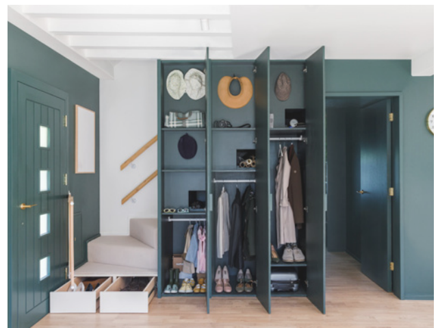
3. Relocated staircase with storage underneath
